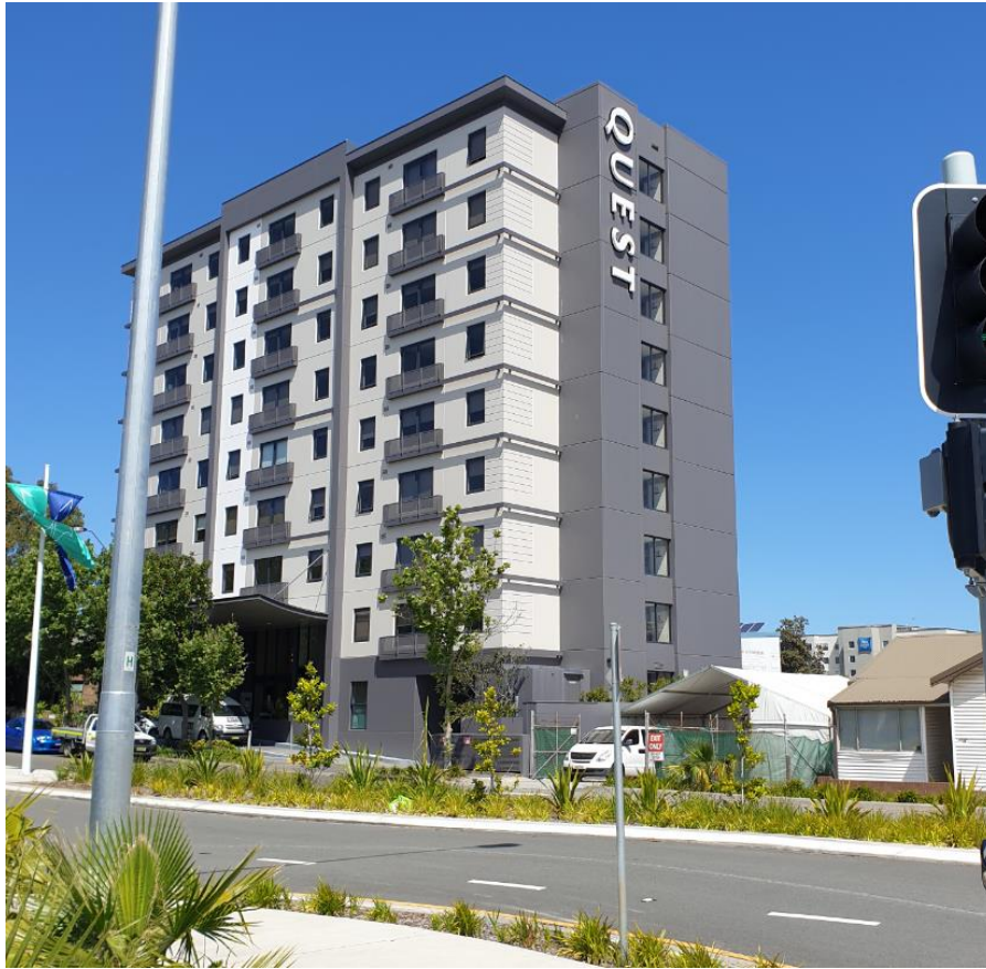
Figure 7. Hotel adjoining at 108 Robey Street
