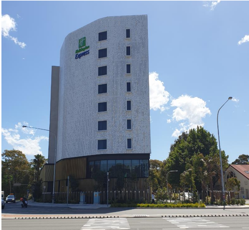
Figure 5. Hotel site opposite at 2-8 Sarah Street
