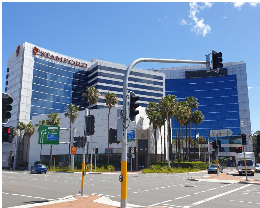
Figure 6. Hotel and office site opposite at 241 O'Riordan Street
